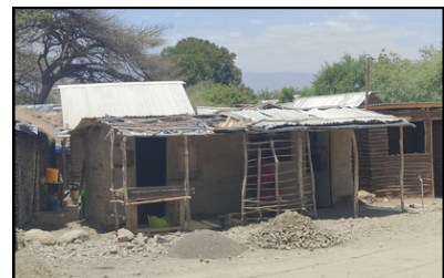
Figure 1: Enkajis with corrugated iron roofs
